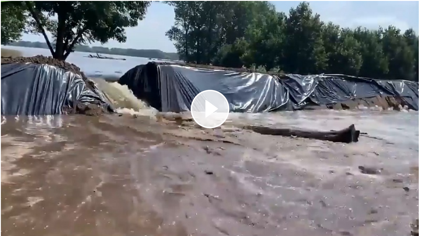
Nooddijk gebroken in Horn. © Dumpert
